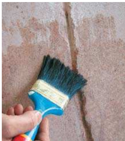
(2) Application of RIALTO PRIMER (interior walls) or RIALTO STABILIZER (exterior walls)
