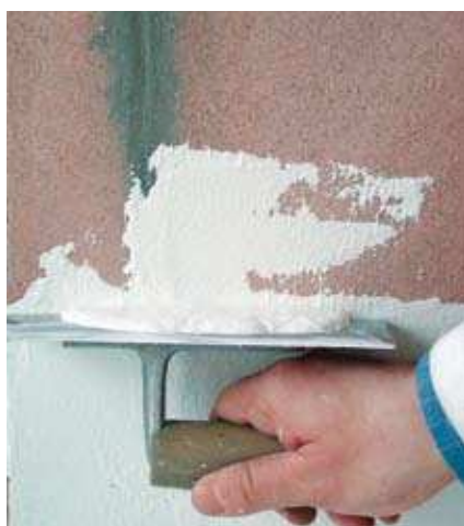
(4) Total leveling treatment with a coat of RIALTO RASELAST
